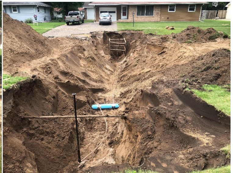
Water service replacement just before backfilling on Edgewood Ln
