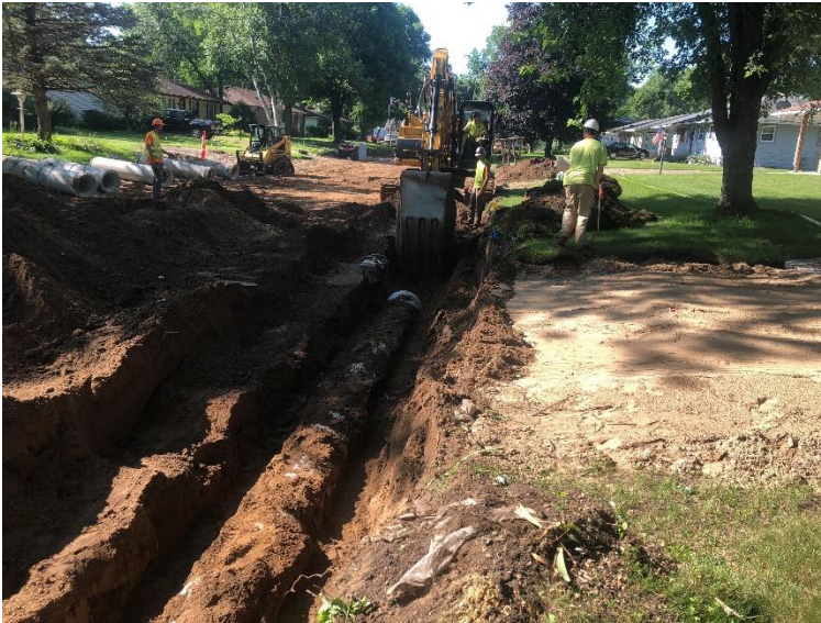
Storm sewer main installation on Edgewood Ln
