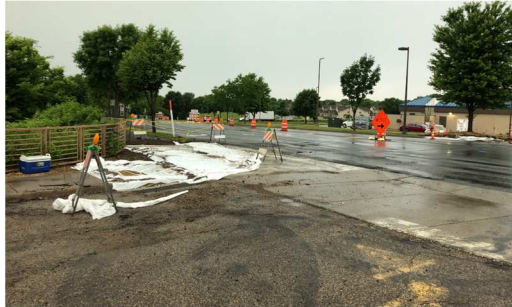
Above Center: Protecting fresh concrete pour from rain...
