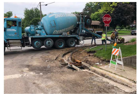
Above Right: Pouring concrete curb on Tyler St
