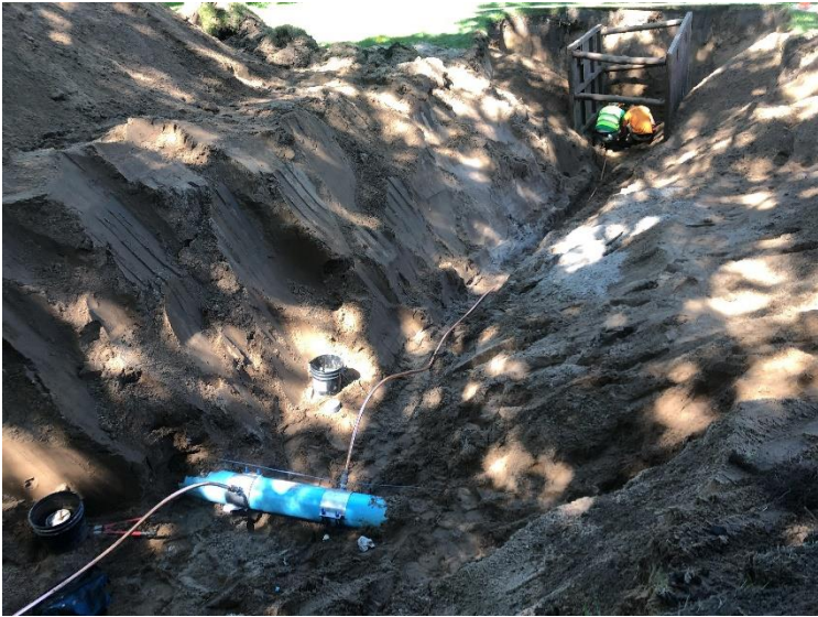
Water service line replacement in progress on Ridge Lane
