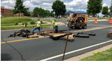
Above Left: Removing Bituminous....
