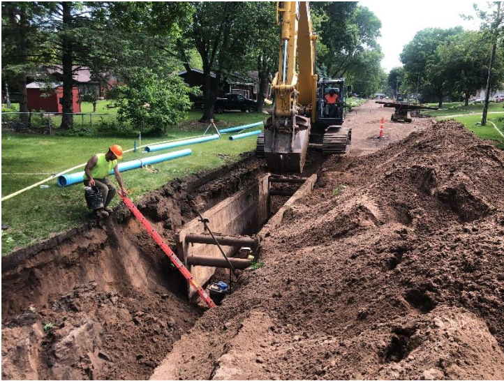
Water main replacement on 21 st Street
