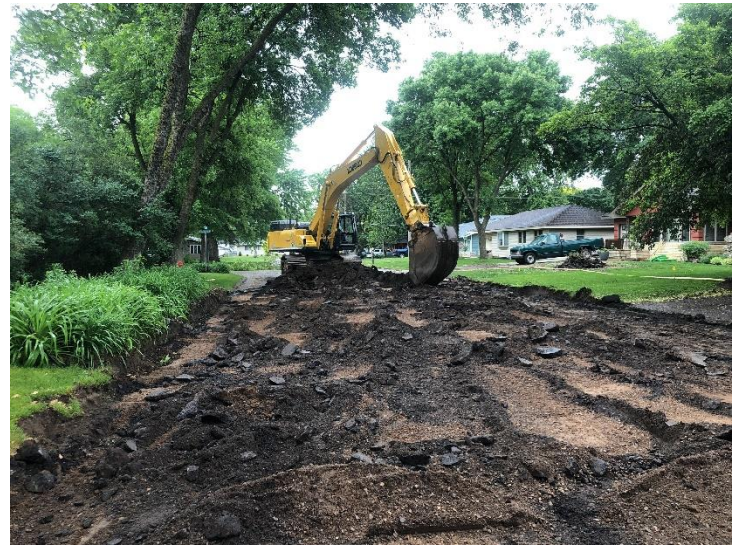
Pavement and curb removal on 21st Street
