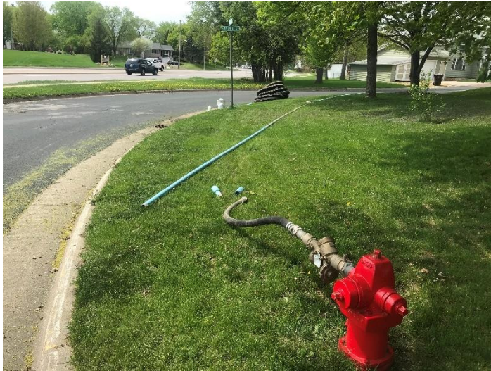
Examples of temporary water main installation
