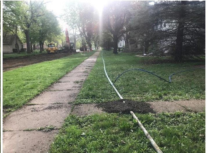
Examples of temporary water main installation
