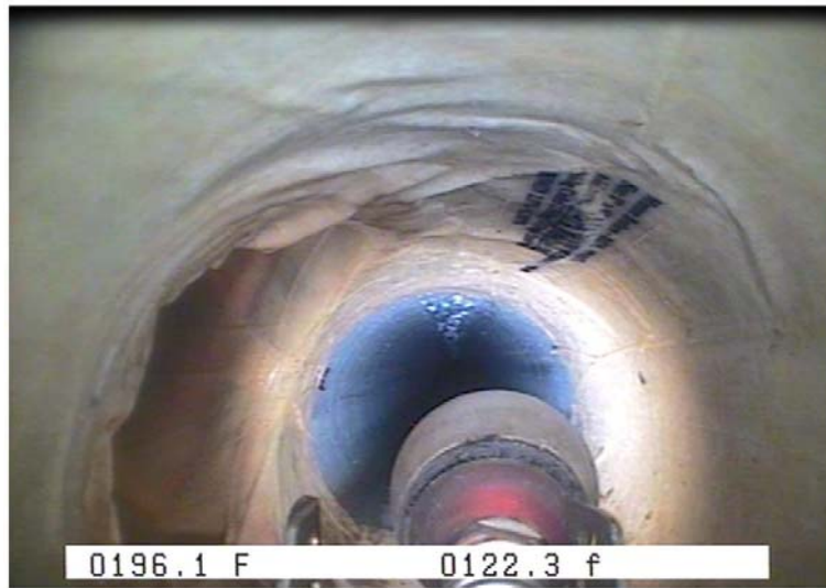
Main Line and Service AFTER Lining
